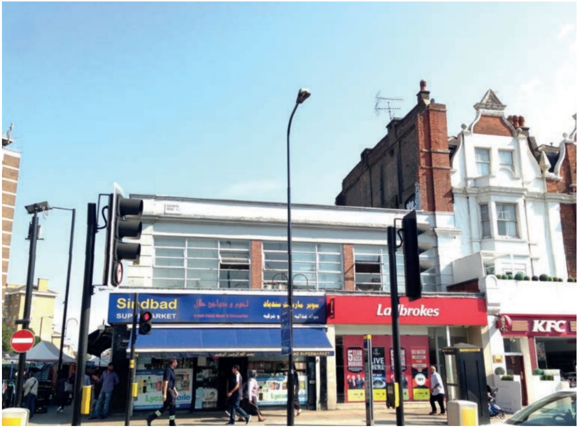
382-386 Edgware Road and 125-127 Church Street (Site A)
