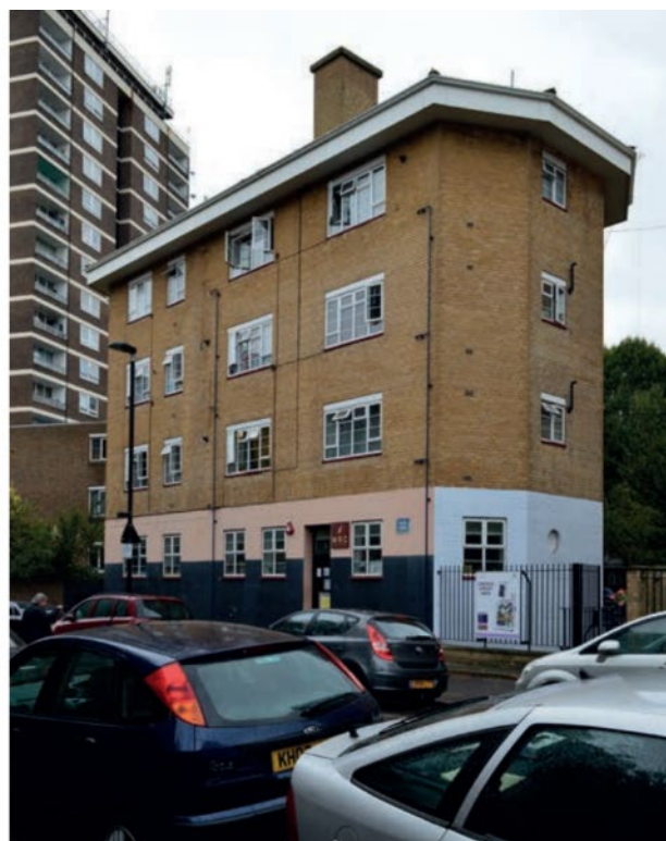
Derry House – Penfold Street(Site C)
