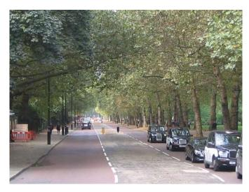
Birdcage Walk, the lighting on the right hand side (path lighting) is of a height where it sits below the tree canopies, however the lighting on the left (road lighting) being higher is now within the tree canopies, affecting the performance of the installation and communication of the control system.
